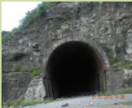
Tunnel T-2 abandoned
