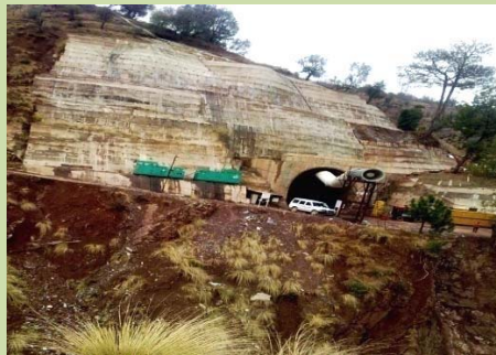
Portal P-1 of T -43 abandoned
