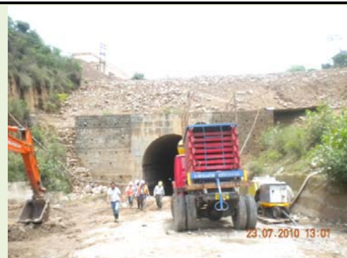
Reconstruction work of T1 portal 2 in progress
