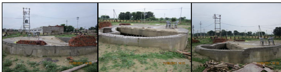
Sumpwell under construction in Sector-6C, Vrindavan Yojna No.1, Lucknow
