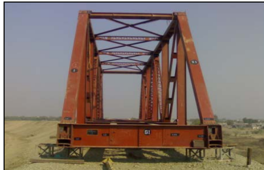
Open web girder
