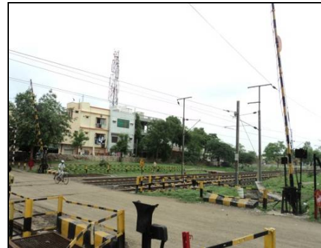
LC No.1B at Nagda (WR) not closed even after commissioning of ROB
