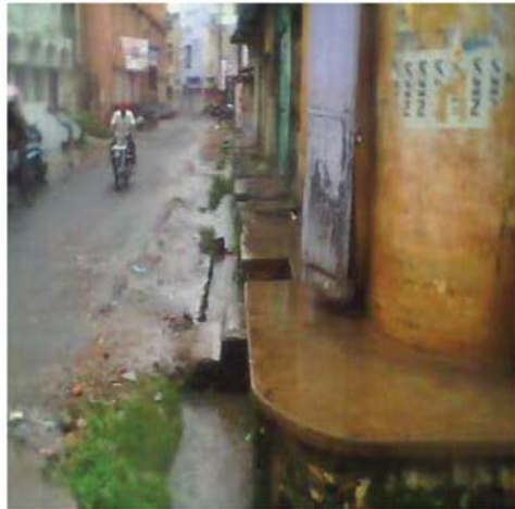
Open drainage system in the area of MC, Gondia
