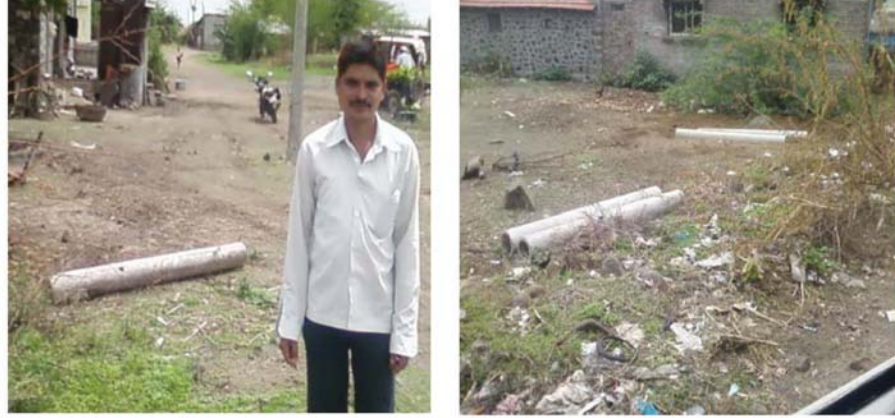
Pipes for compartment bunding lying scattered in the villages
