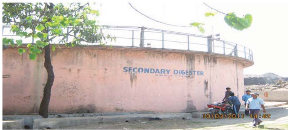
Secondary Digester of the STP at Adharwadi
