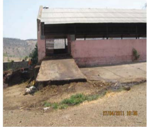
Abattoir releasing effluents and solid wastes
