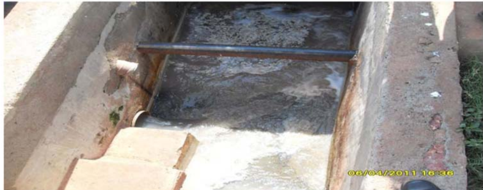
M/s. Gadre Marine Export Pvt. Ltd., Ratnagiri, Flow meter at inlet point not installed
