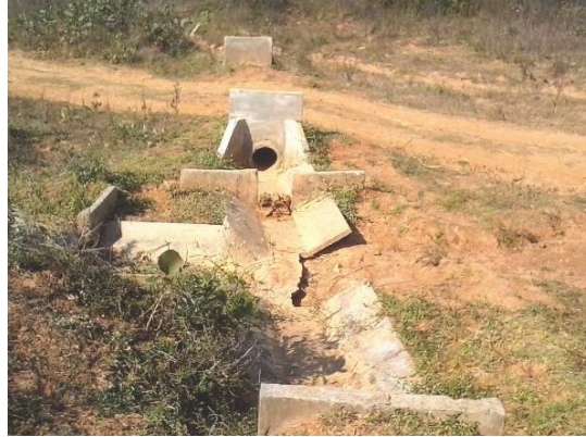
A view of lined water course near Waraseoni Sub-Jail in District Balaghat, where RCC lining work was stated to be done.
