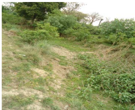
Blocked Field Drain
