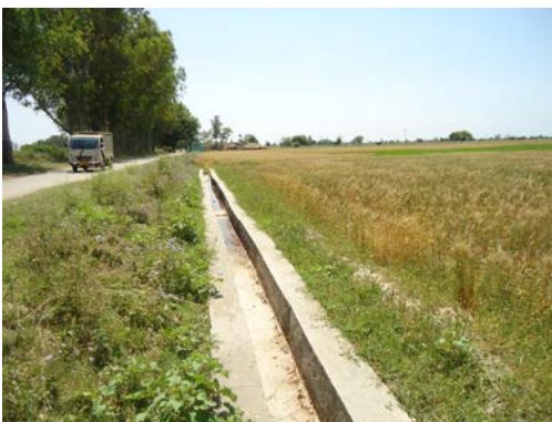
Plum Concrete Field Channel (RS Pura/December 2010)
