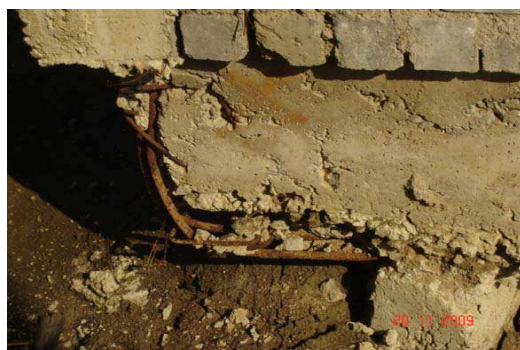
Picture showing eccentricity of Column at Mathpurena site – BSUP Raipur (The compressive strength of concrete work was found 111.15 kg/sqcm against the standard of 200 kg/sqcm.
