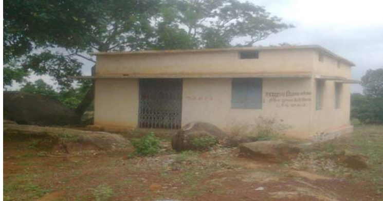
Idle dispensary building in village Ranpur (Block-Jashpur)
