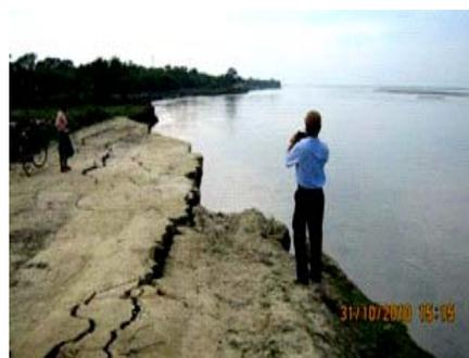
**Eroded (breached) newly constructed embankment**
