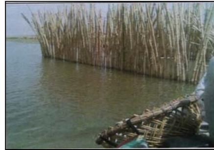
**Bamboo made submerged vanes
