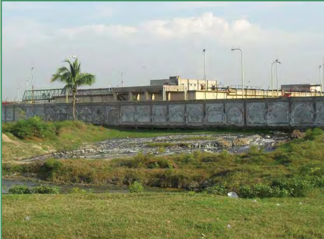
Effluents flowing along the boundary of CETP
