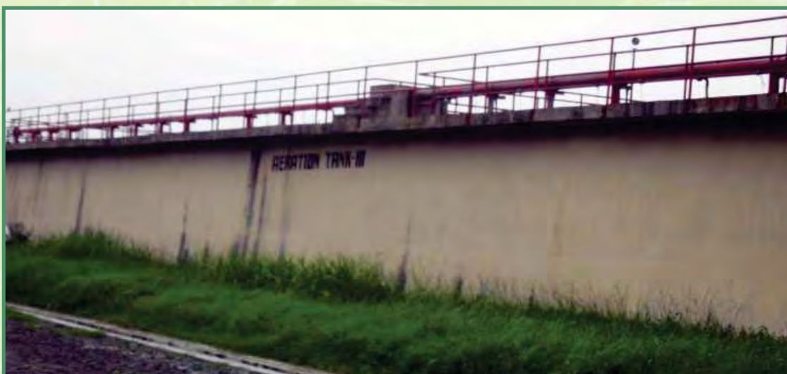
Defunct aerator tank
