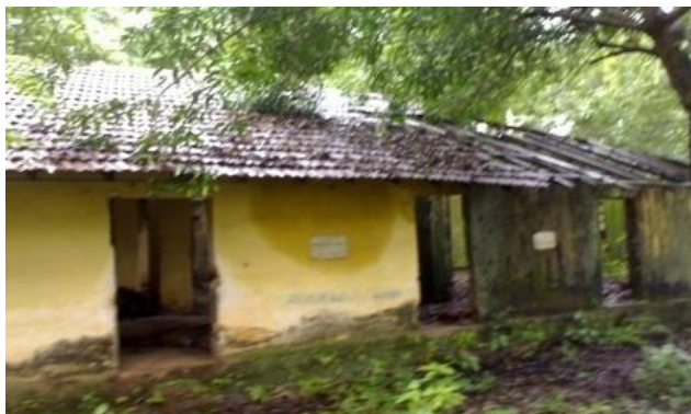
Dilapidated condition of leprosy hospital
