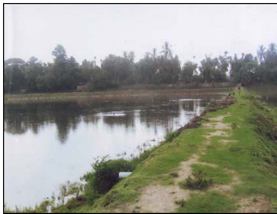
Reclamation of RM Dighi at Udaipur
