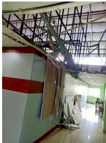
Pic 3.11: Ceiling of corridor at 1 st Floor leading to DM's chamber
