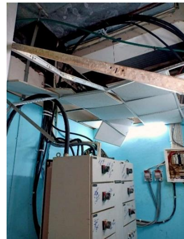
Pic 3.12: Collapsed false ceiling of the Electrical Unit at ground floor of the Auditorium
