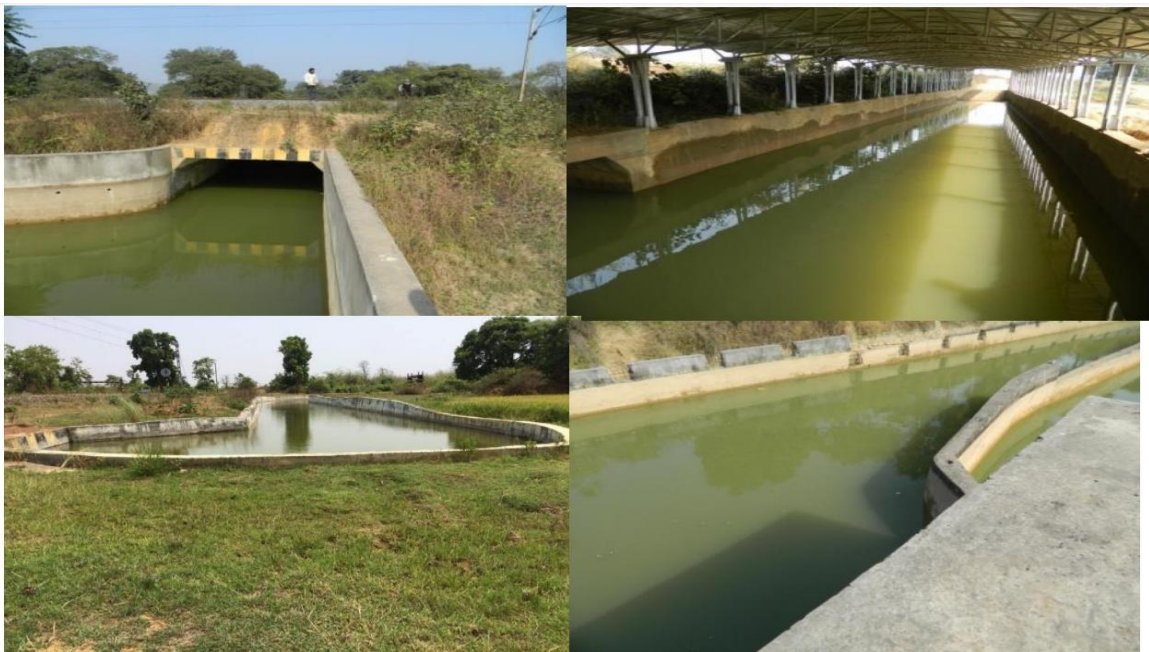
Clockwise - LHS 295 (Dongha Dhakel-Raigarh), LHS 286 (Bhikharimal-Raigarh) and LHS 294 (Parsada-Raigarh) has Water accumulation with mud; and LHS GCF-49 full of water up to the brink-looking like swimming pool and could not be commissioned due to water logging
