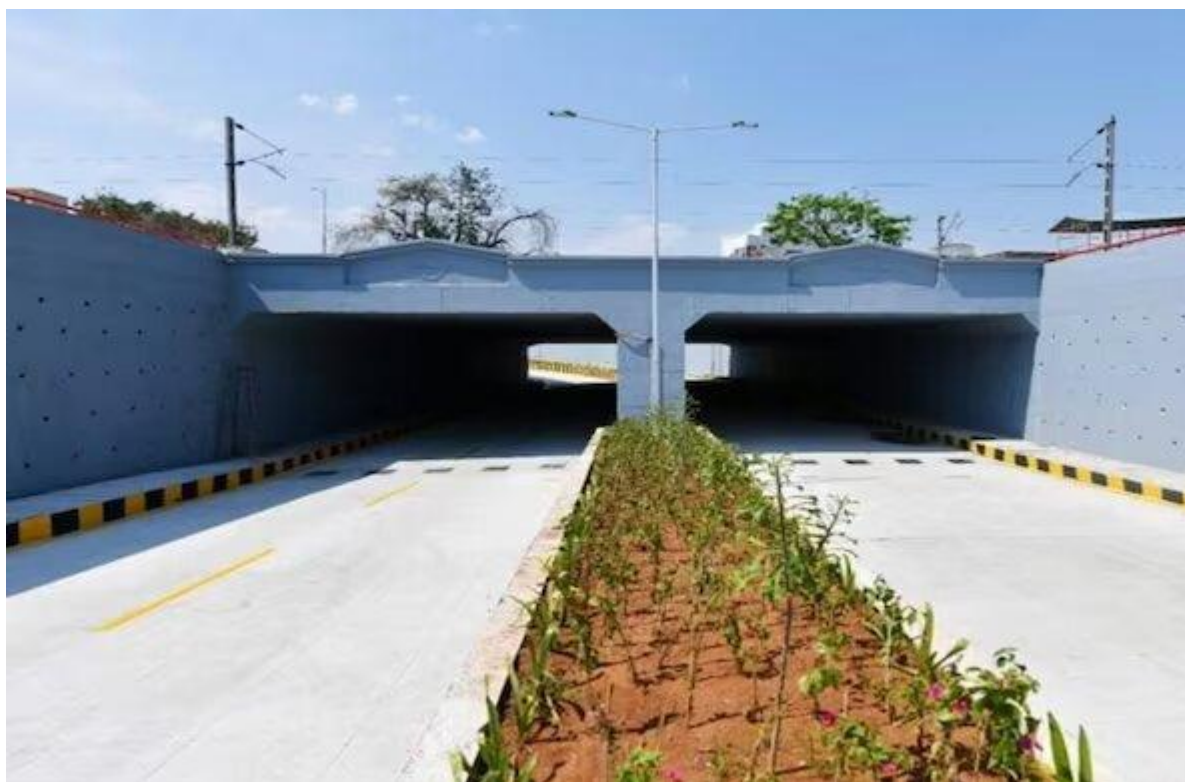
Road Under Bridge
