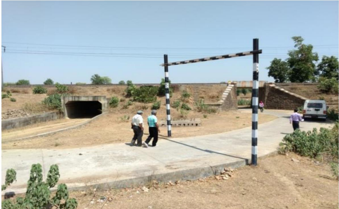
LHS at LC No. AB-24 and diversion RUB
