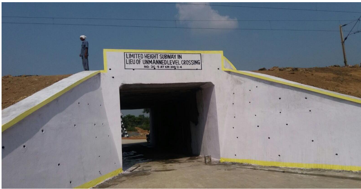
Limited Height Subway
