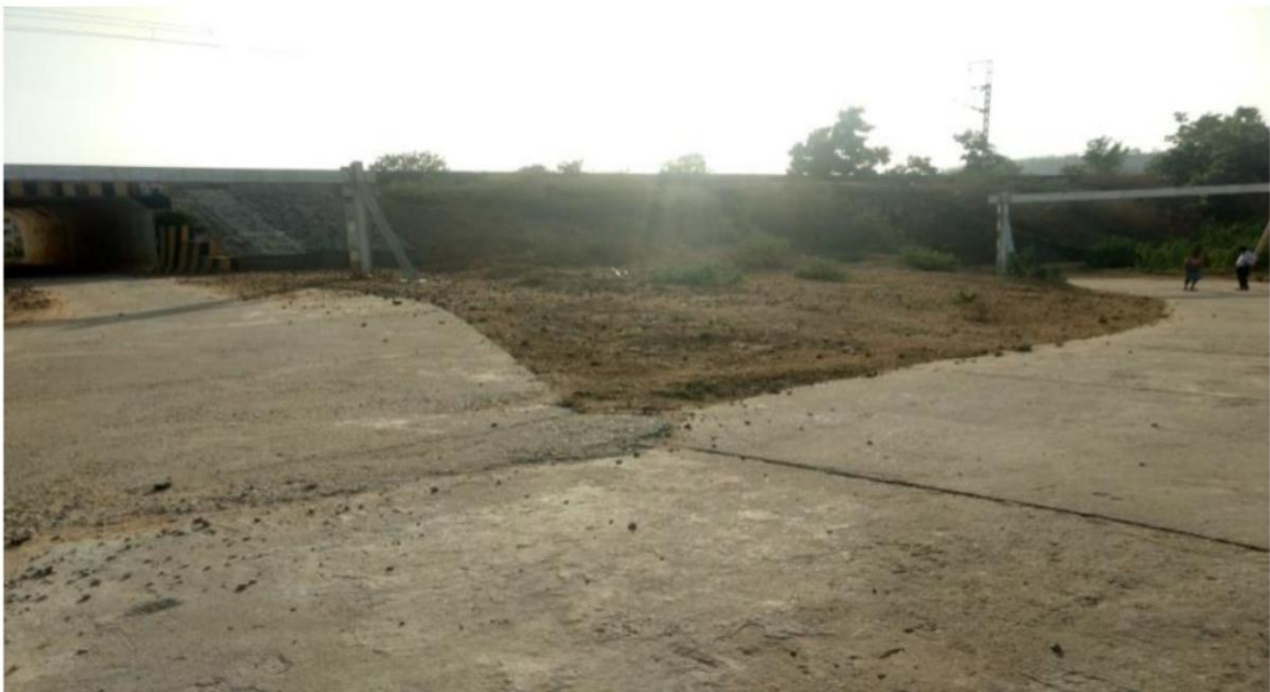
LHS at LC No. AB-35, LHS and diversion RUB
