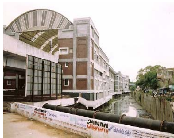
Thirumailai station adjacent to slum clusters and canal
