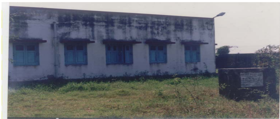
Photograph showing the non-functional Kalinagar Central Hostel
