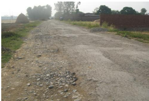
Shimla-Pistaur-Kuraiya Road (KM - 4)
