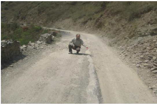
Chakrata-Lakhamandal Road (Km. 24)
