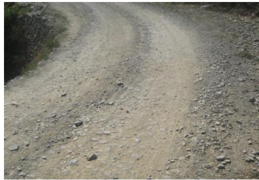
Chakrata-Lakhamandal Road (Km. 36)
