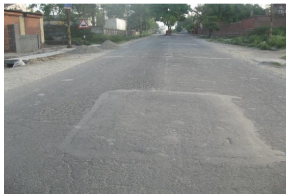
Niranjapur Bend to Shimla by-pass Road (KM 1.2)
