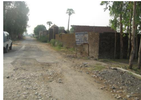
Shimla-Pistaur-Kuraiya Road (KM - 4)
