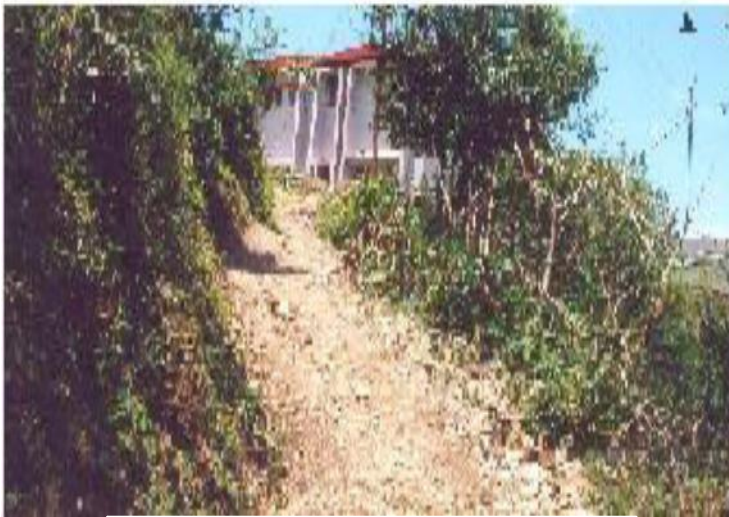
CHC building at Thatyur without approach road
