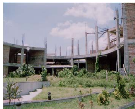
Incomplete structure of Cultural Museum
