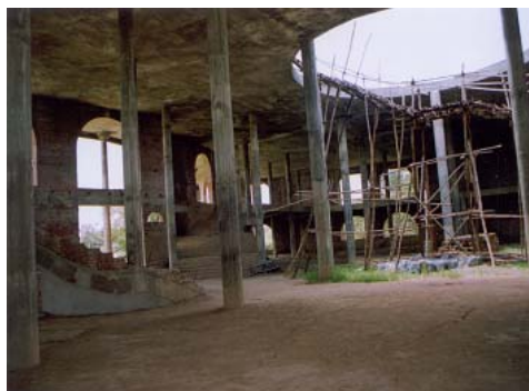
Incomplete structure of Irrigation Museum
