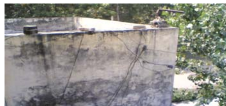
Boys' Hostel at Chhauchh, Lakhimpur
