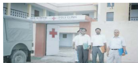
Hostel at Kanpur Dehat occupied by a Polyclinic
