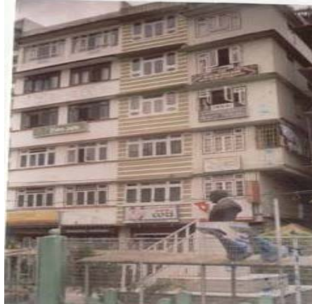
Adjacent buildings without proper gully at MG Marg
