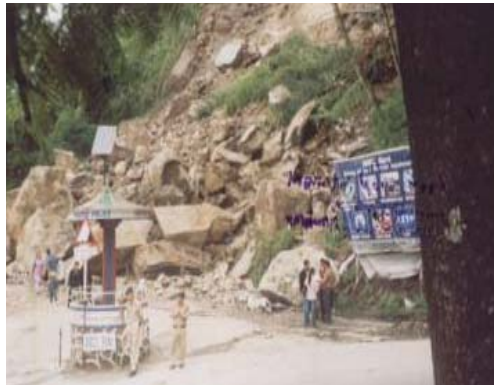
Landslides due to absence of guard wall in hill side of roads at Amdo Golai
