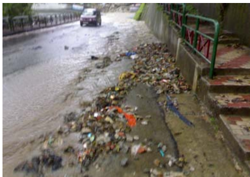
Inadequate drains leading to overflow of water in NH 31A
