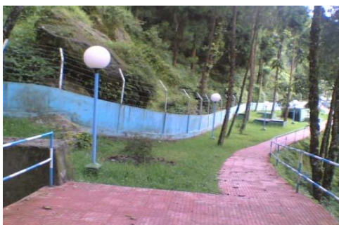
Beautification works in Selep Treatment Plant: Laying of tiles etc.
