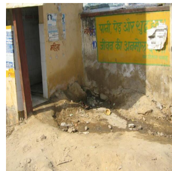
Drainage at Chaksu
