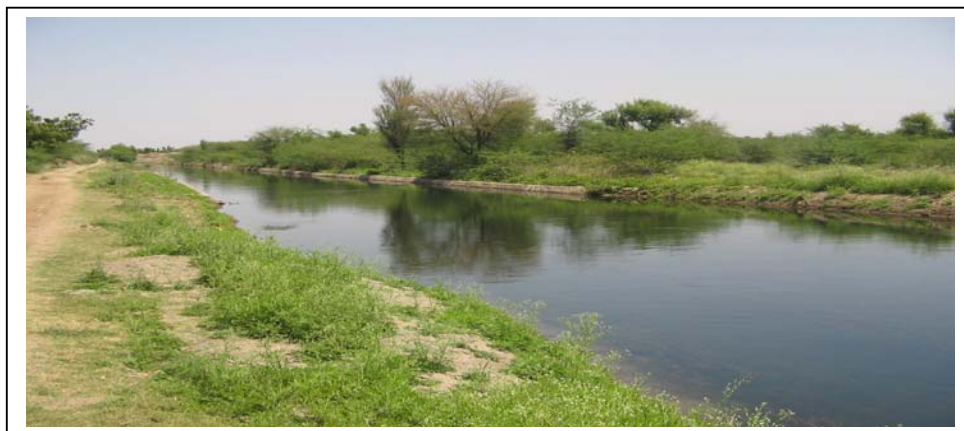
Dismantled old lining of Jawai main canal, Sumerpur
