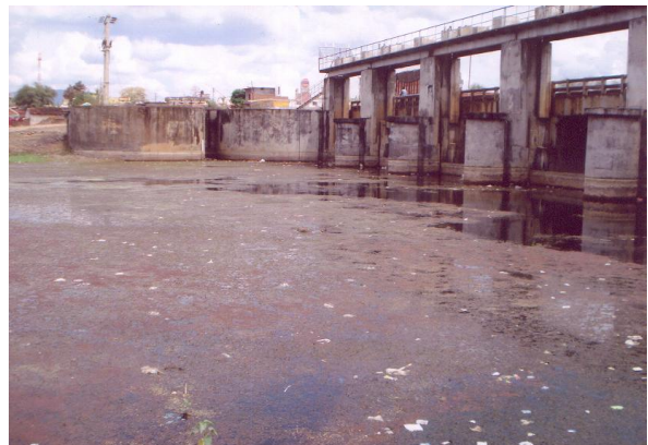
Completed Barrage (Stage-I)
