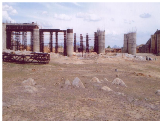
Incomplete Stage II works
