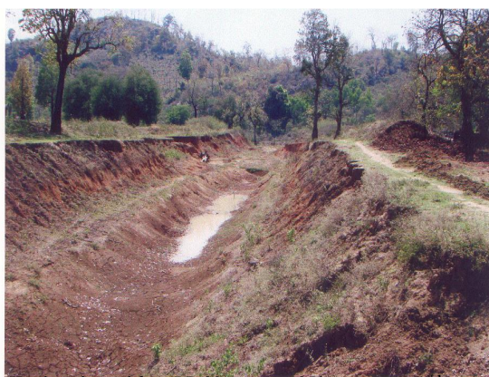
Head reach canal from RD 00 metre to 1250 metres upto 1 st berm
