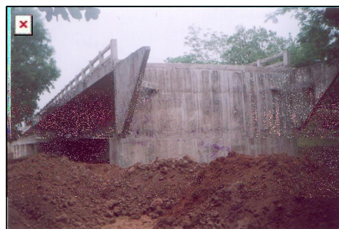
HL Bridge without approach road
