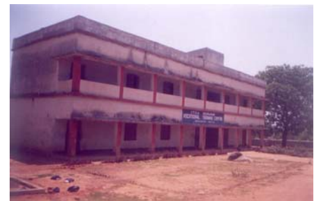
Newly constructed Vocational Training Centre at Naranpur (Keonjhar ITDA) lying unused
