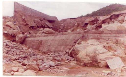
Chute Spillway of Bhagalati Irrigation Project
