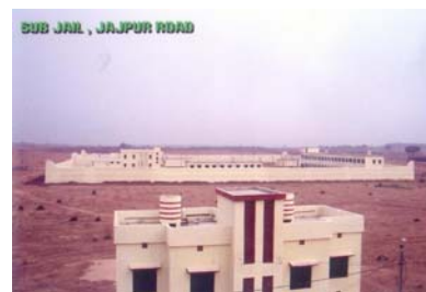
New sub-jail and staff quarters at Jajpur Road lying unutilised
