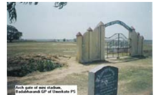
Prohibited work-Arch gate of mini stadium of Badabharandi GP, Umerkote PS
