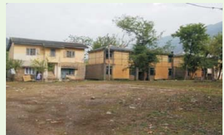
Dilapidated condition of residential facilities for staff at CHC Sunni.
