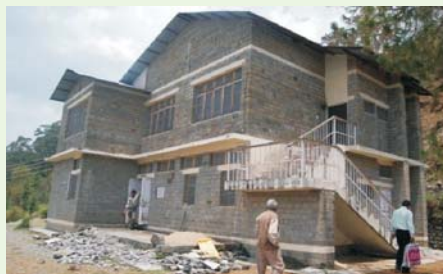
PHC Naldehra under repairs
