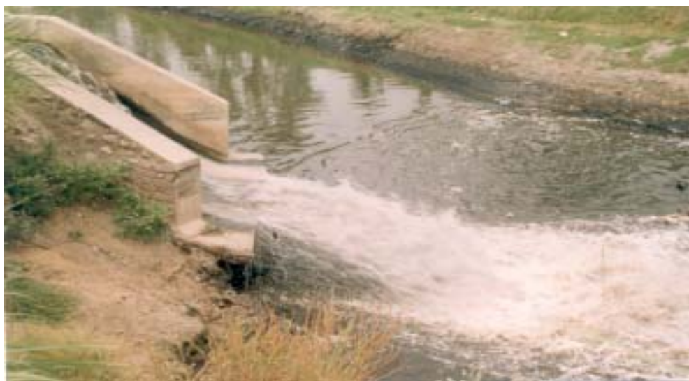
Treated effluent from 25 MLD, STP at Camp area Yamunanagar coming out through effluent channel and falling into a Nallah running near the STP which flows into WJC
