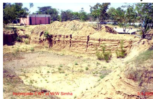
Incomplete second clear water tank at water works Seehma
