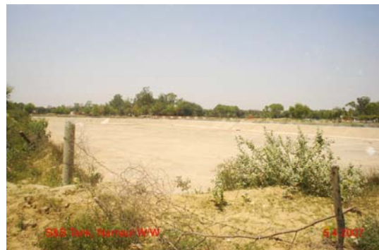
Empty storage and sedimentation tank at Narnaul water works
