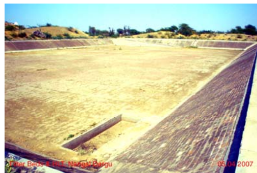
Empty storage and sedimentation tank at Nangal Dargu water works
