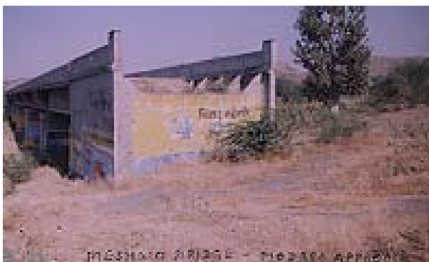
MESHWO BRIDGE MODASA APPROACH
