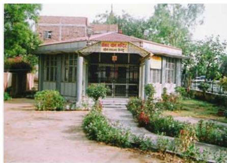
Public Library cum Utility Centre at Hari Nagar
