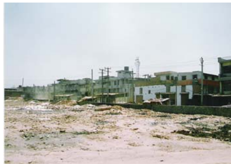
Boundary Wall & MS Grill to enclose a park in A-Block, Wazirpur Industrial Area
