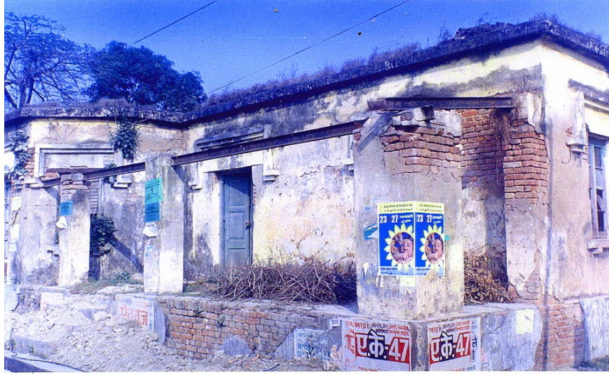
Building of PHC, Lalgang, Vaishali
