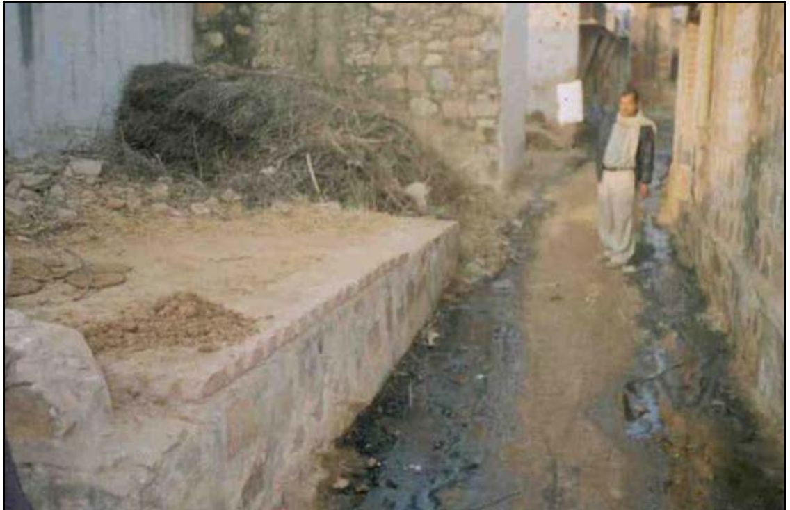
A view of damaged CC road of village Indravali
