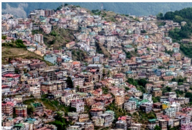
Haphazard construction of buildings in Cemetery area of Sanjauli, Shimla, Himachal Pradesh
