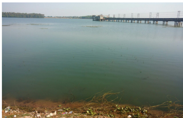
Rukka dam (Design Capacity-170.50 MLD) (14/03/2017)
