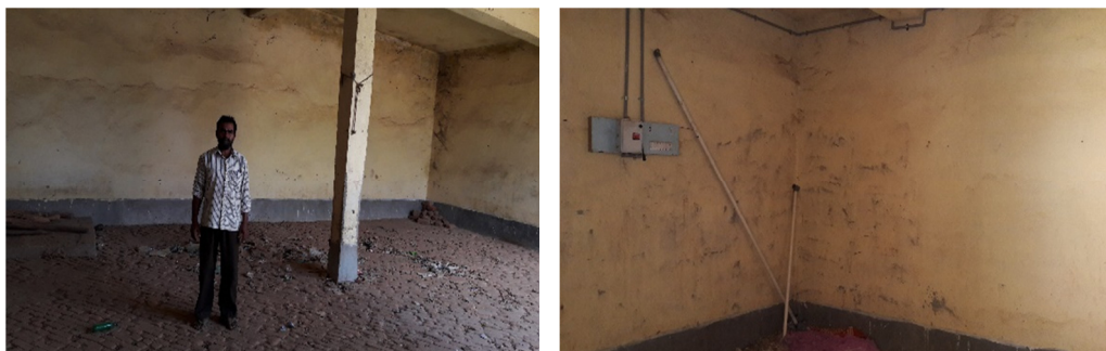
Flooring and plumbing was not done in respect of works at Sarauni, Godda (as on 4 August 2016)
