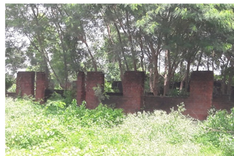
Photograph (12 August 2016) showing PB constructed upto lintel level and abandoned (Polpol, Palamu).
