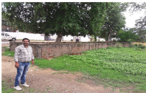
Photograph (12 August 2016) showing shops constructed upto plinth level and abandoned (Nawatoli, Palamu).
