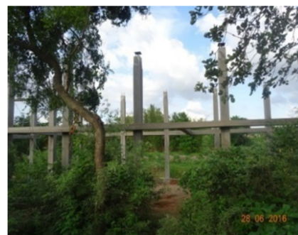
Incomplete Karm shed, Deoghar
