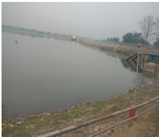
Kanke dam (Design Capacity-19.50 MLD) (19/03/2017)
