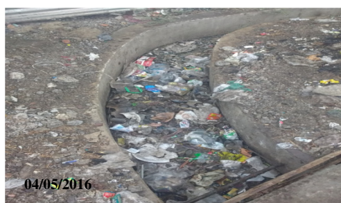
Open drain choked by garbage at Bhuiyandih, Jamshedpur
