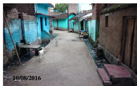
Silt deposited in drain, near Railway Station, Sahibganj
