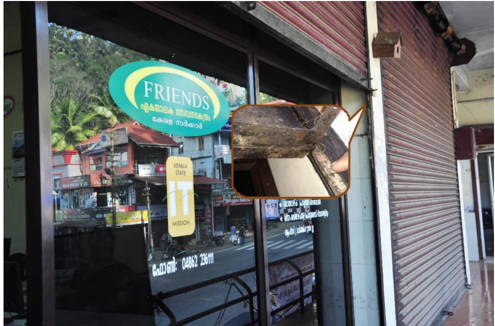
Picture depicts view of Idukki Centre, where the steel shutter cannot be closed. The shutter channel is blocked with wooden logs to prevent collapsing of the damaged steel shutter. Inset picture displays a wooden log used as blockade.
