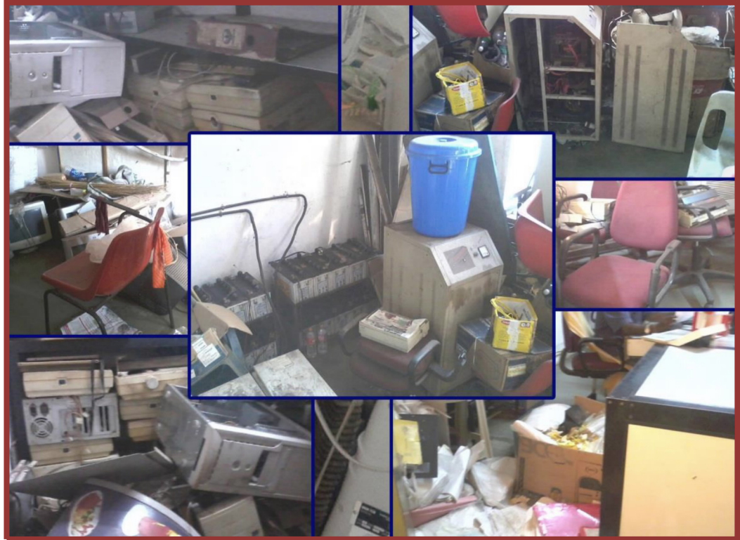
Picture shows dumping of scrap over the UPS, battery and near the counters in Thiruvananthapuram and Malappuram Centres.
