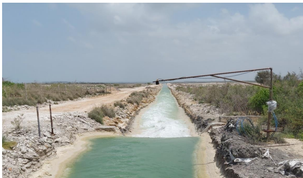
Figure 4.1: Treated wastewater being discharged through open channel at marine outfall point in Gulf of Kachchh at Mithapur
