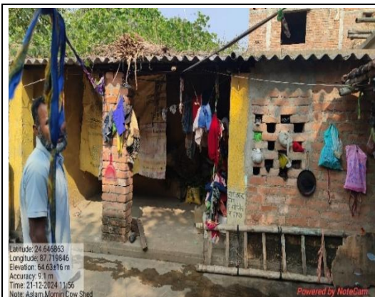
Photograph 6: Cowshed in Pakur district used for residential purpose
