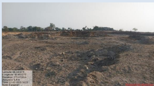
Photograph 3: Construction of pond in land of Vijya Devi at GP Pipardih in Garhwa
