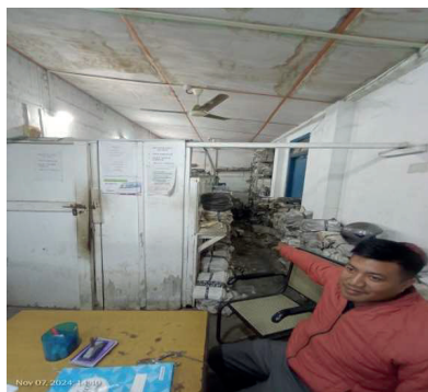
Photograph showing keeping of physical records at the area where frequent waterlogging happens during heavy rainfall (DTO, Imphal West)
