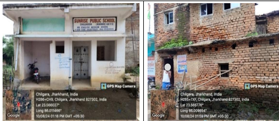
Photograph 2.4 and 2.5: House constructed under PMAY- G used for running a school and old pucca house of the beneficiaries
