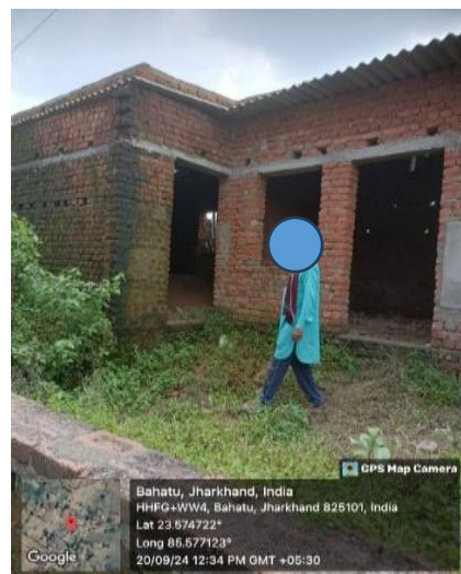
Photograph 2.8: House constructed on CCL land by the beneficiary
