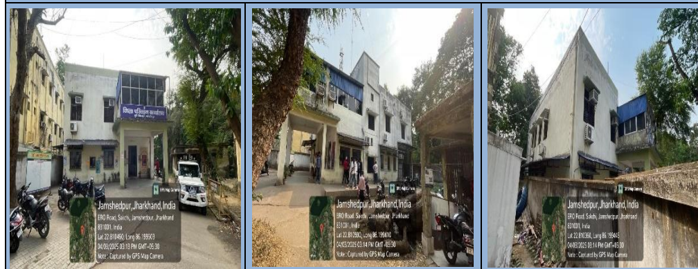
Photograph 2.11: DTO and MVI office, Jamshedpur, functioning in its own building in a newly constructed building in the premises of District Collectorate.
