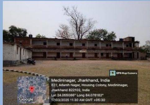
Photograph 2.7 : Driving training school functioning in the premises of an educational institution.
