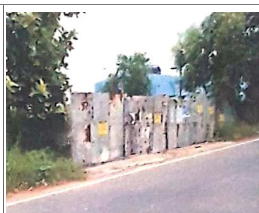
Figure 4.26: Temporary boundary wall of Auditorium, made of old tin sheets and bamboos, in dilapidated condition
