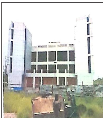
Figure 4.24: Outside view of Auditorium after renovation work
