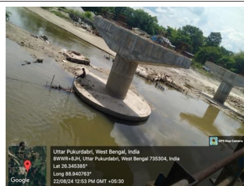
Figure 4.15: Bridge over River Saniajan at Kangratoli on Imigration road under Teesta Bridge Construction Division in the district of Coochbehar
