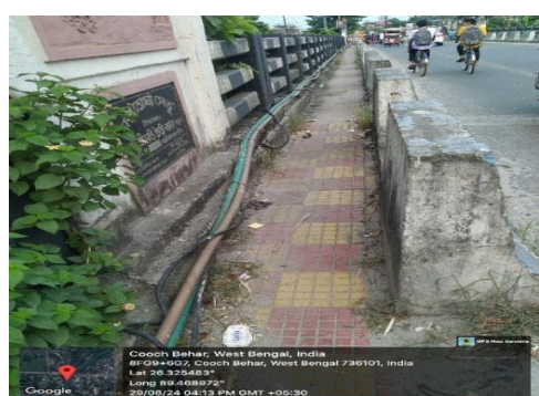
Figure 4.11: Cable line laid in footpath of the Mora Torsha bridge at chainage 2.00 km of Coochbehar Dinhata Gitaldah Road under Cooch Behar Division (PWD)
