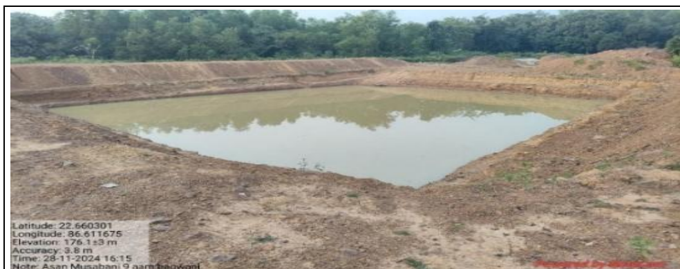
Photograph 2: Pond was constructed in place of mango plantation at Asna GP
