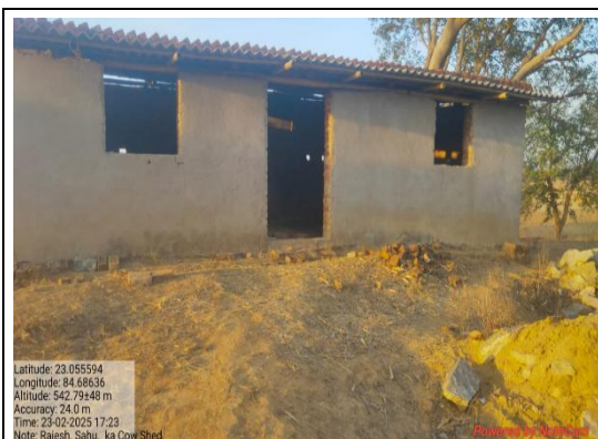
Photograph 8: Cowshed in Gumla district constructed with bamboo and asbestos sheet
