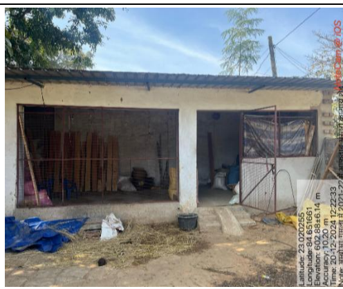
Photograph 7: Cowshed in Gumla district was being used for storage purpose.
