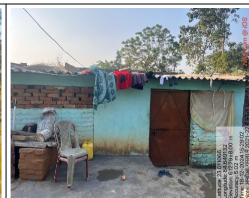
Photograph 9: Cowshed in Gumla district used for constructed with bamboo and asbestos sheet
