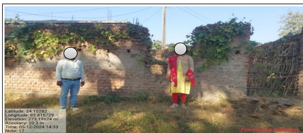
Photograph 1: Incomplete construction of Anganwadi Centre, in Garhwa
