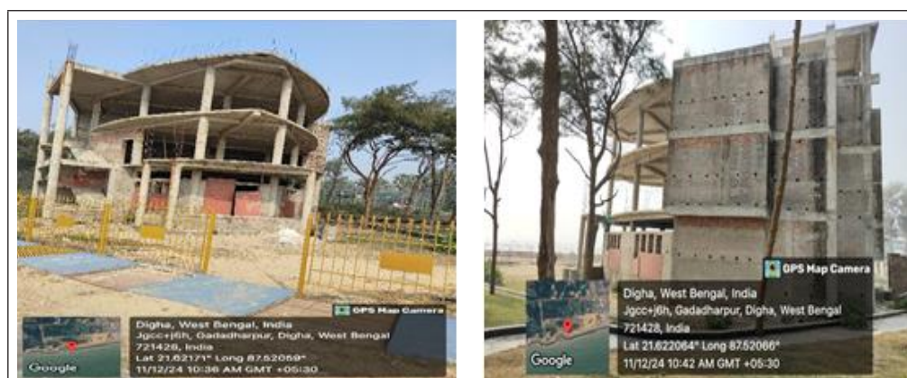
Figure 3.5: Under construction of amenities centre and food court under CRZ area
