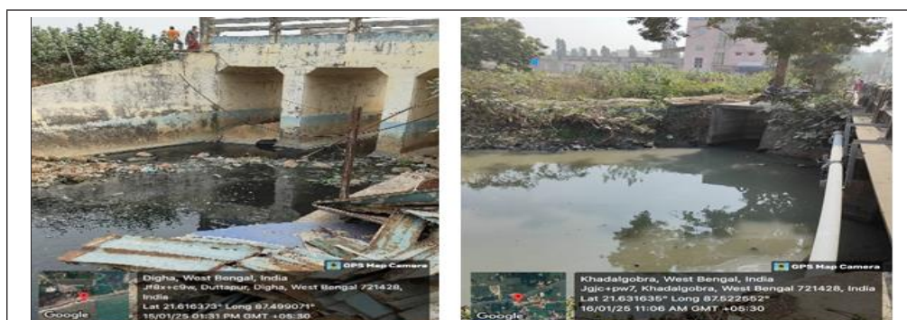
Figure 3.7: Discharging of polluted water into sea without treatment at Jatranala, New Digha and Mohana, Old Digha
