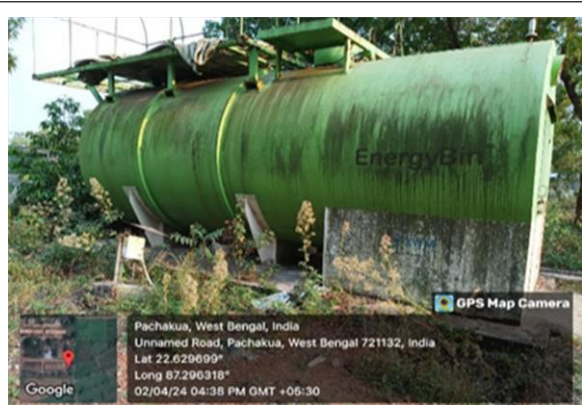
Figure 2.5: Bio-methanation plant, Salboni
