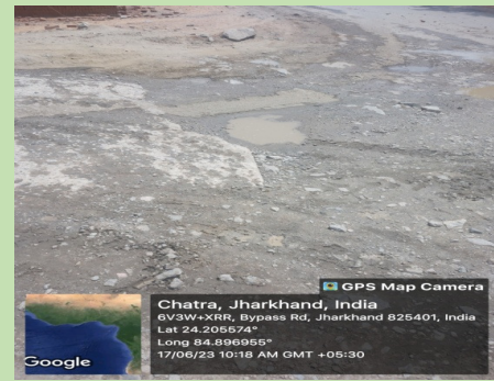
Picture-4.37: Showing completely damaged PMGSY road in mining area (due to plying of heavy mining vehicles) in Chatra and Palamu districts
