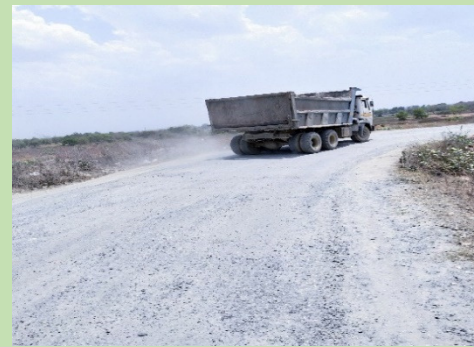
Picture-4.37: Showing completely damaged PMGSY road in mining area (due to plying of heavy mining vehicles) in Chatra and Palamu districts
