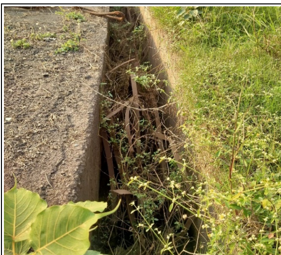
Figure 6.9: Baling hoops lying inside a drain at Durgapur Warehouse
