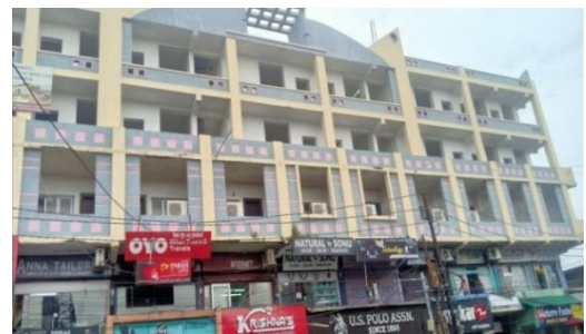
View of Mayuree Tower at Satyanarayanpur
