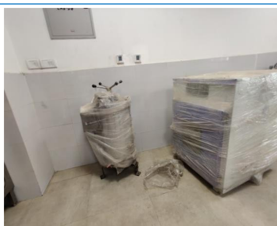
Picture 11.30 Machines in packed and uninstalled condition in Quality Control Lab (Noida Campus)
