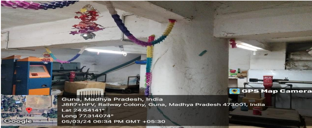
PMS system was not installed at Guna Station of West Central Railway
