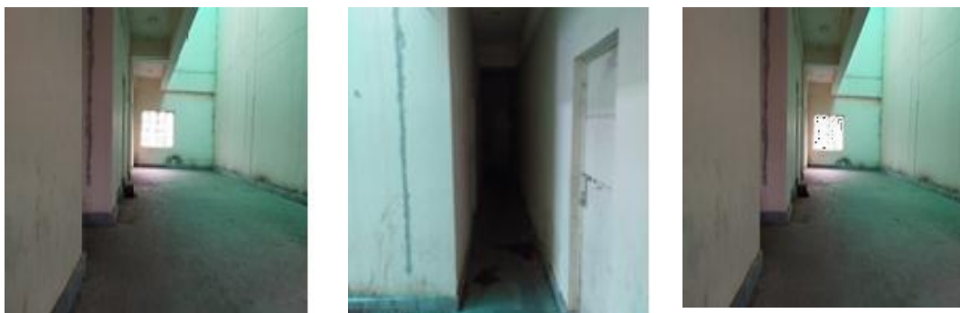
Photograph No. 3.1: Images showing the unutilised facilities in the SEC Building
